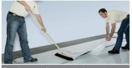
Fig. 3: pulling the protective film to one side and pressing on, preventing any blisters
