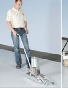
Fig. 4: welding the membrane with the alwitra solvent welding machine
