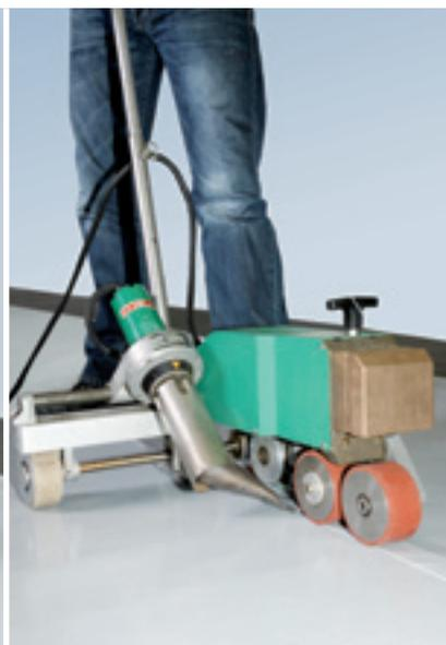
Fig. 5: welding with the hot air welding machine
