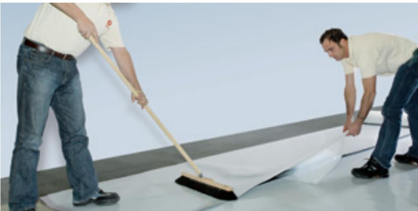
Fig. 3: pulling the protective film to one side and pressing on, preventing any blisters
