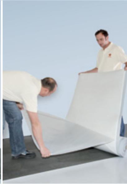
Fig. 2: peeling off the protective film
